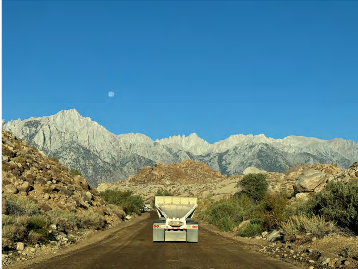
Image 1. Sta 652+00 Bk (looking West), hauling in borrow
