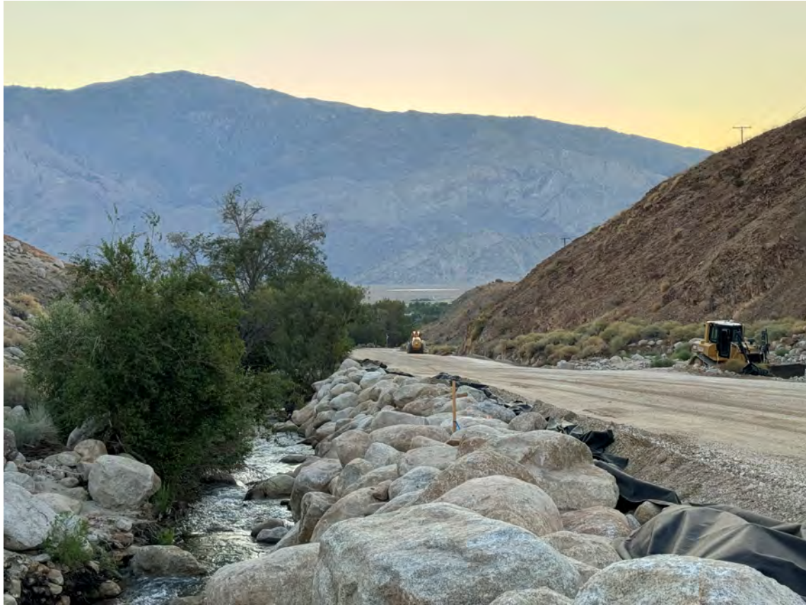
Image 7. Riprap Embankment Slope Protection - Complete Station 655+50 Ahd (Looking East)
