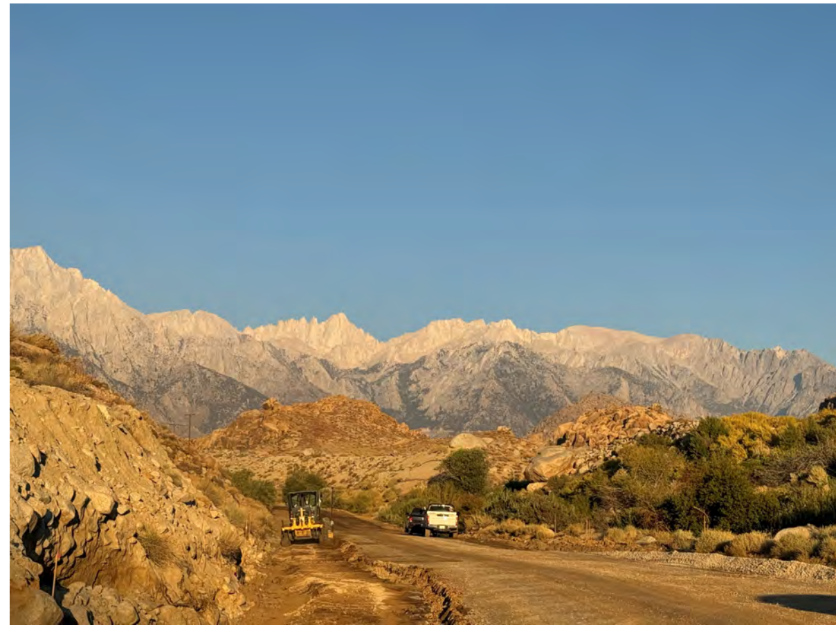
Image 3. Embankment Construction - Station 667+60 Bk (Looking West)
