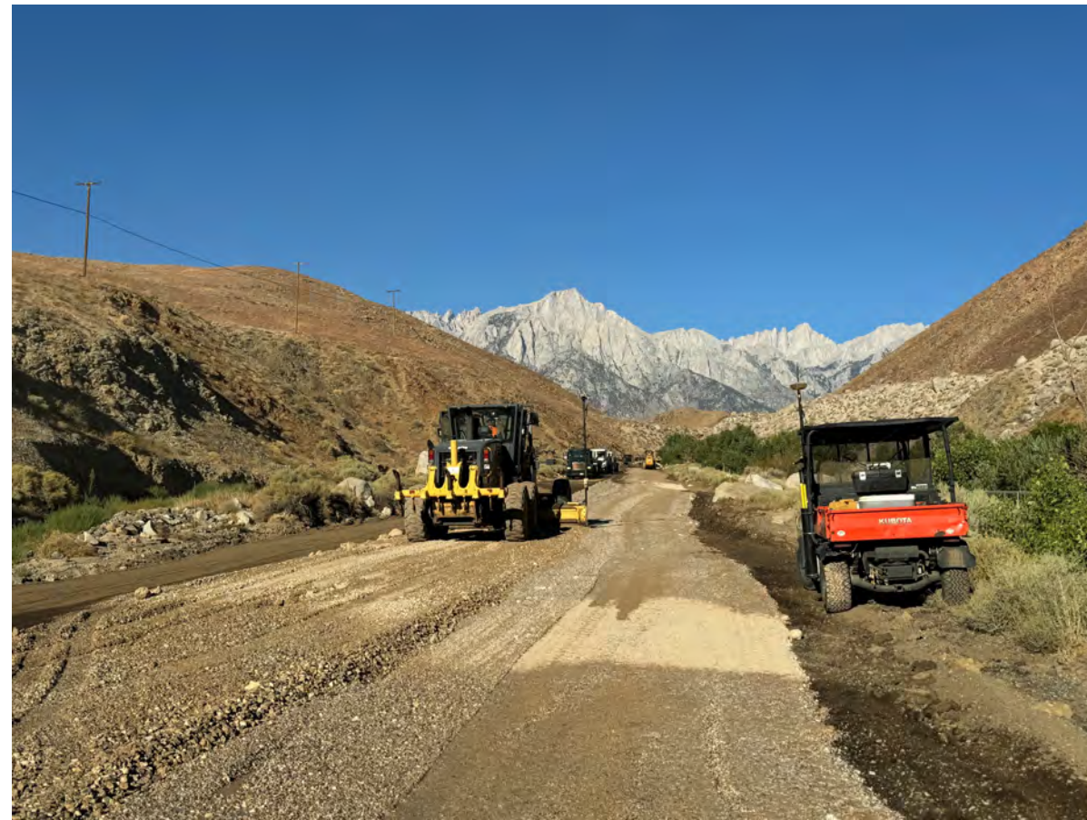
Image 4. Embankment Construction - Station 670+00 Bk (Looking West)
