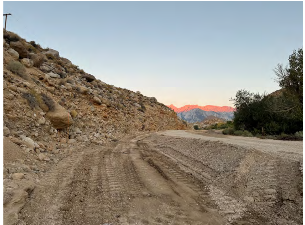
Image 8. Embankment Construction - Sliver Fill Station 621+00 Bk (Looking West)
