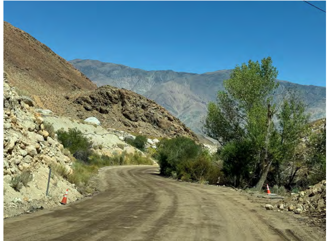
Image 2. Sta 621+00 Ahd (Looking East), Embankment construction
