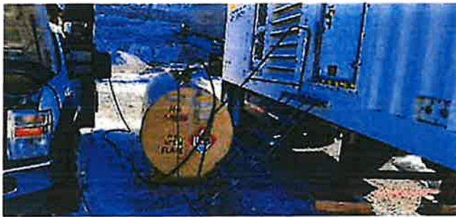
1000 - gallon fuel tank
