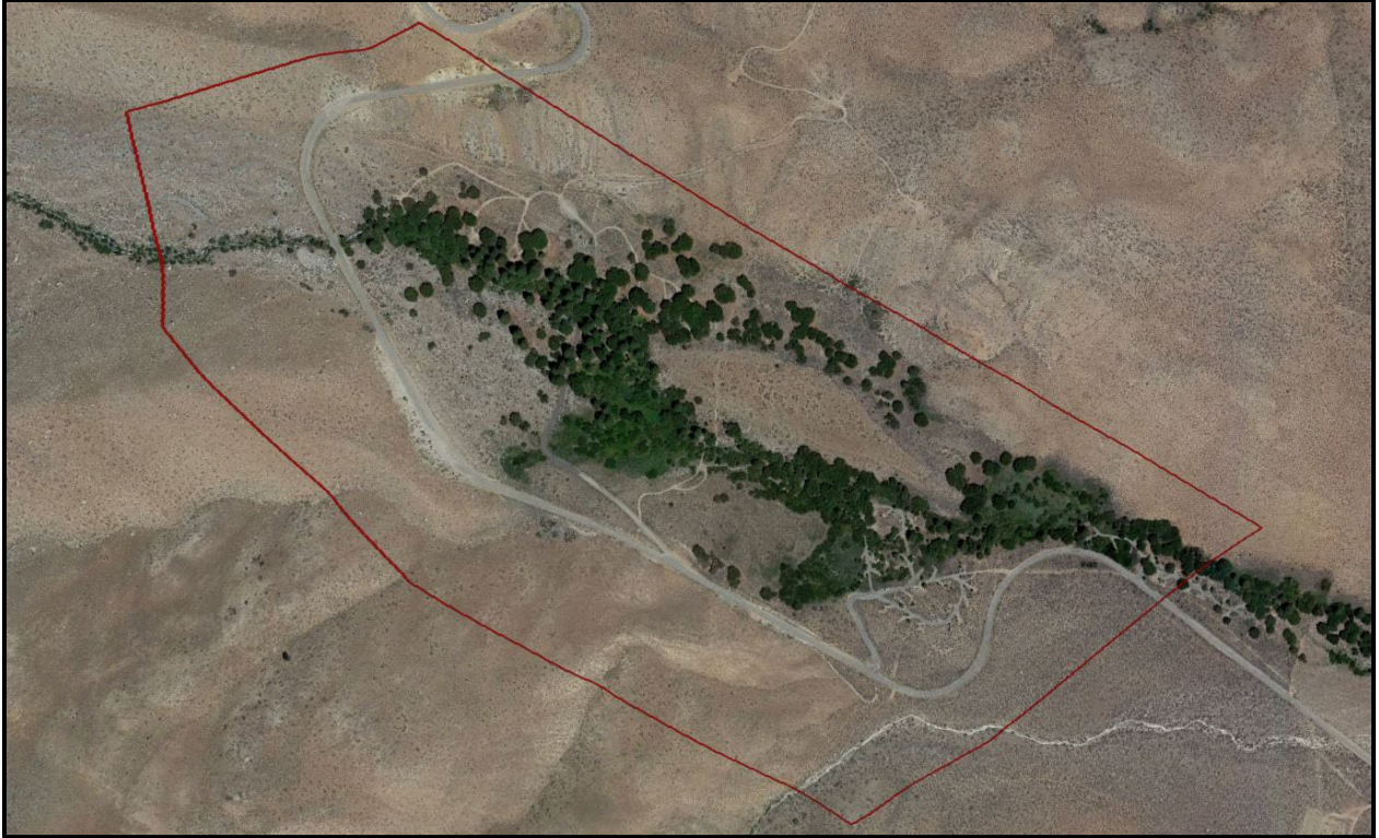
Figure D.2. Cabins are surrounded by shrubs, heavy riparian vegetation, and timber and have limited defensible space. The red boundary is the community boundary.
