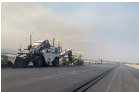
Image 14. Paving operations on Runway 12-30
