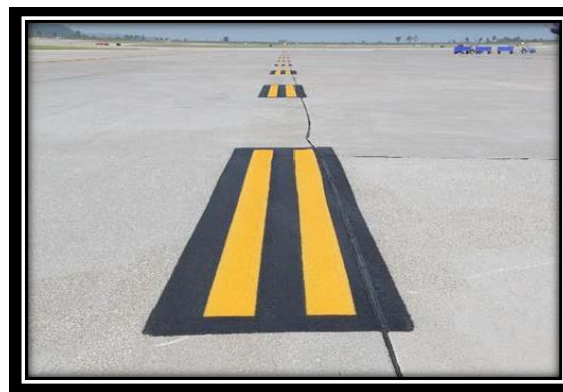
Image 5. Taxiway Edge Marking
