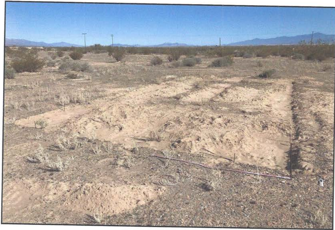
PHOTOGRAPH 7 Excavated Pad with Associated Rebar, Looking North-Northwest
