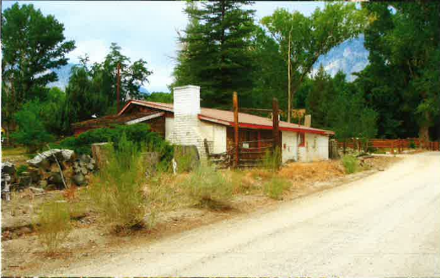
NORTH EAST SIDE OF HOUSE OFF OF BIRCHIM LANE.
