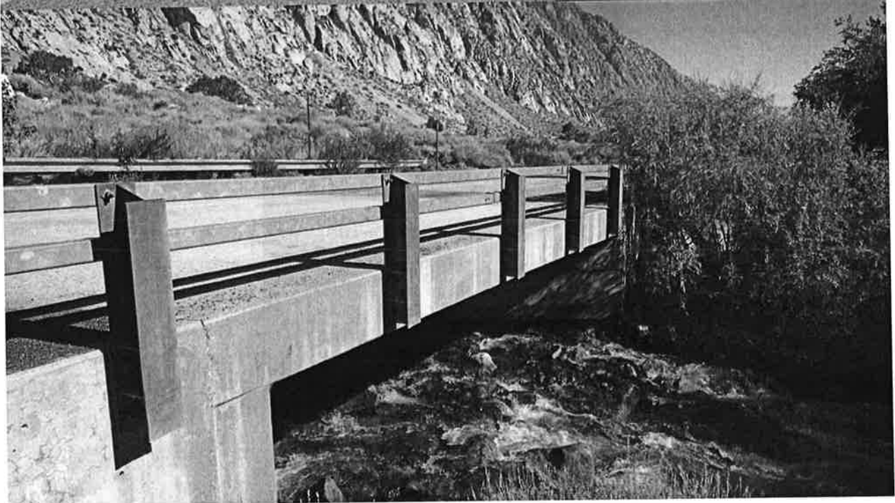
Site 2: Upper Location – Pine Creek Road
