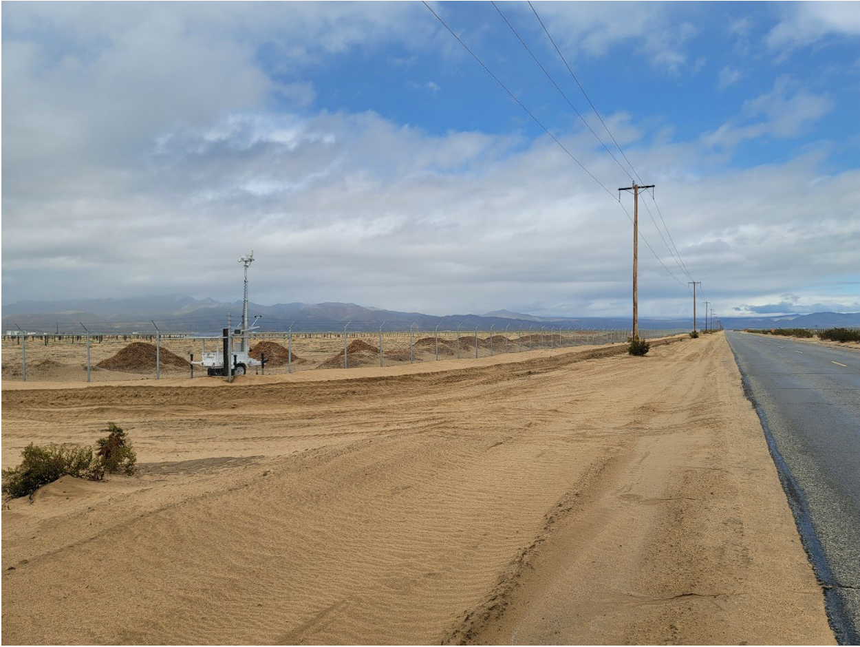
March 21, 2023 Photos of windblown sand at solar facilities near California City right adjacent to Neuralia Road. Apparent mitigation measures here appear to include scaping away of the dust outside of the fence.
