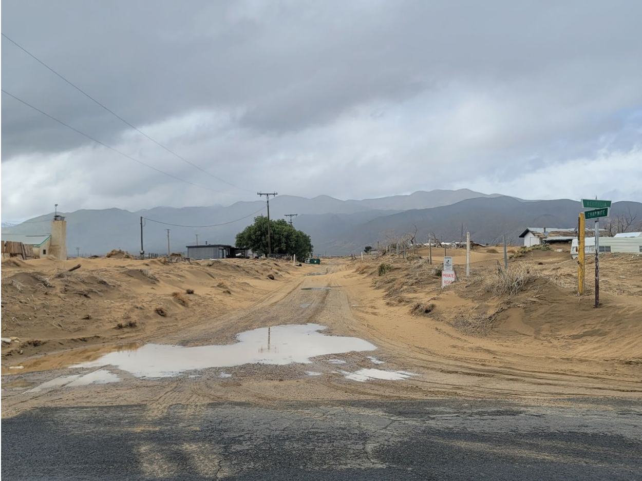
Another Photo. The solar facility can be seen at the end of the road in the picture. Note massive sand accumulation.
