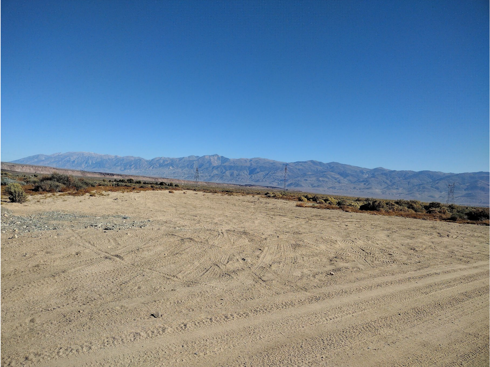
Damage off Tungsten City Road 2023
