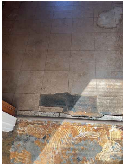
vinyl squares in radio room, including mastic
