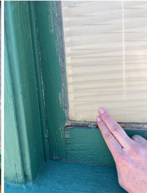
West side of the building
