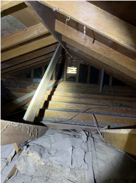
In back room
