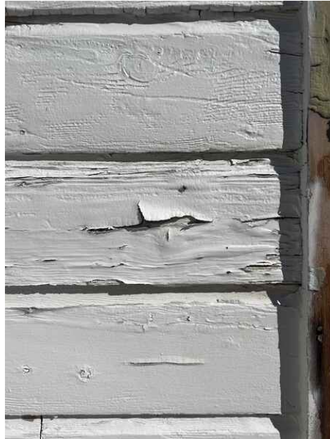
cladding paint--all layers, south side
