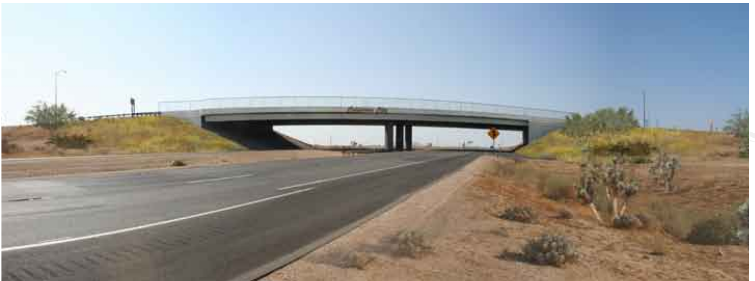
California City SR 14 Interchange After Enhancements
