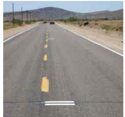
Example of Speed Bars Along Highway
