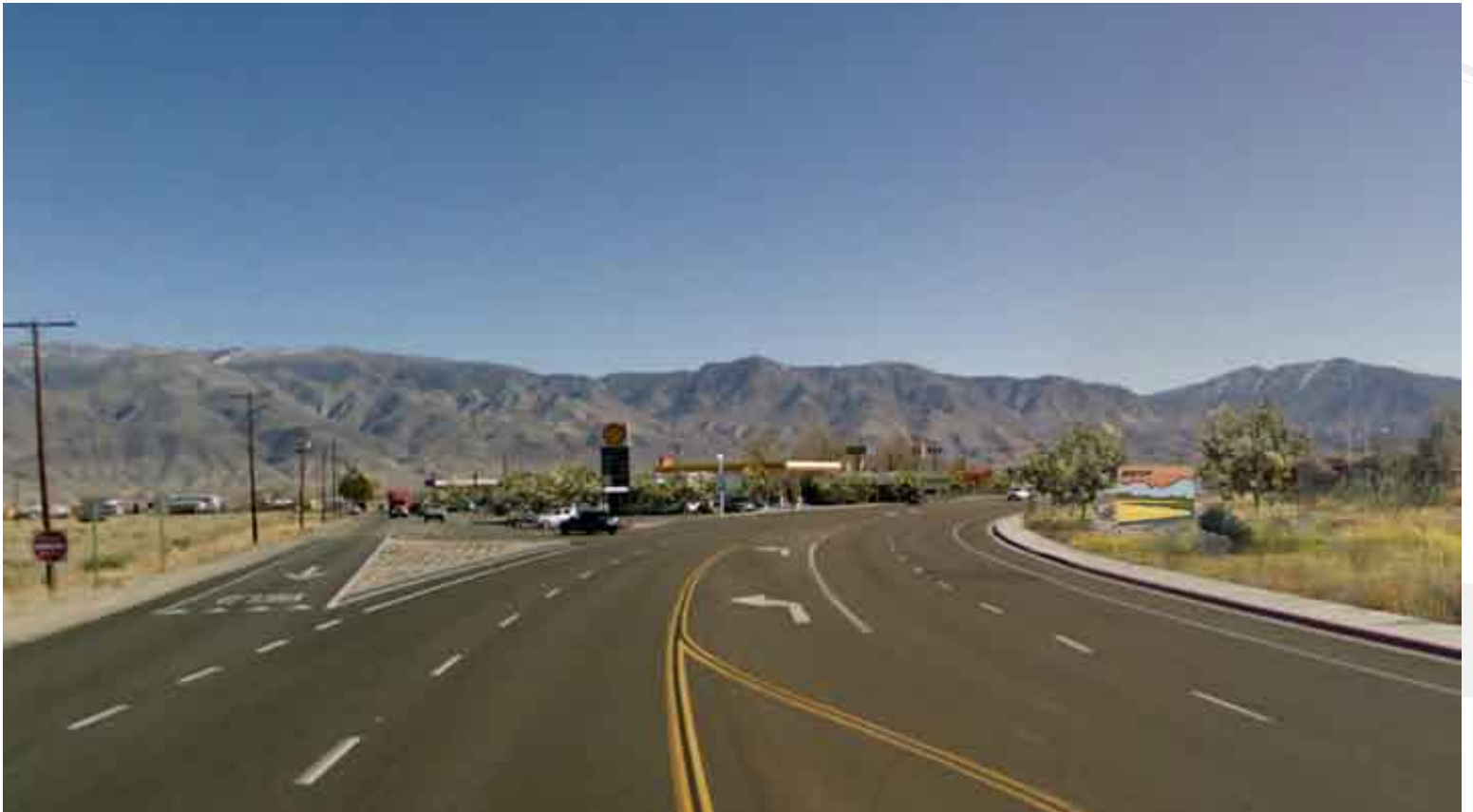
Bishop Entry at Wye Road Intersection After Enhancements
