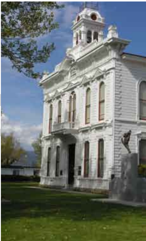
Bridgeport County Courthouse
