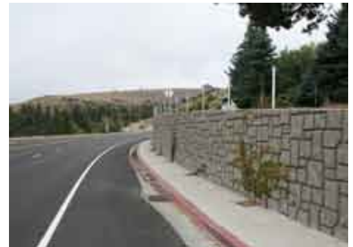
Lee Vining Streetscape with Enhanced Retaining Wall
