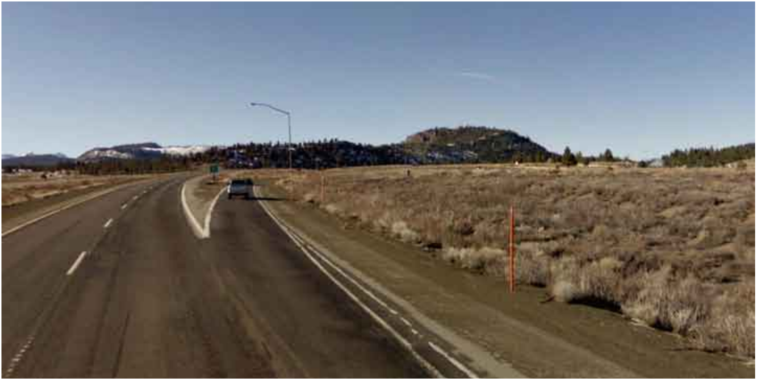
Mammoth Lakes Interchange Before Enhancements
