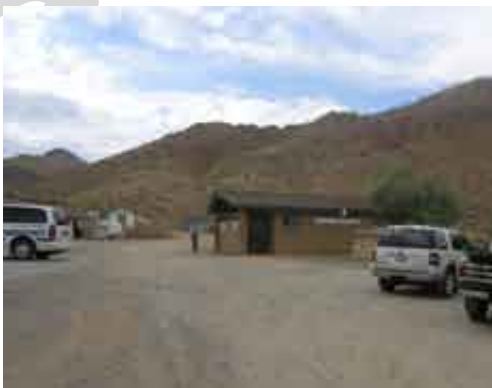
Public Restrooms at Park in Walker
