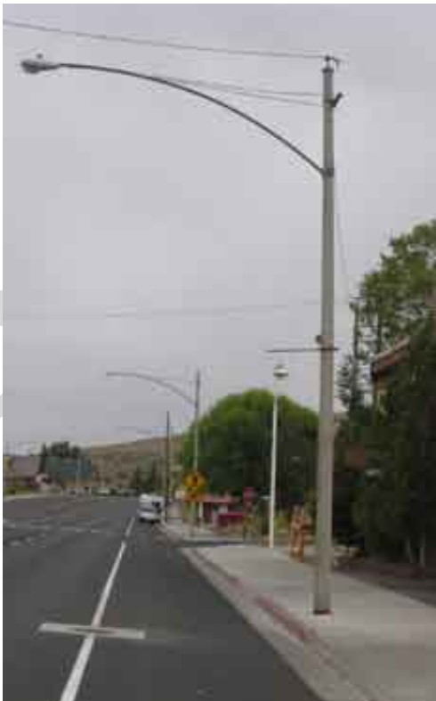
Lee Vining Streetscape with Multiple Curb Cuts Which Limits On-Street Parking
