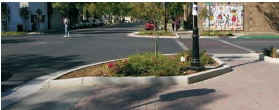
Tighter, shorter turning radii reduce traffic speed and shorten pedestrian crossing distances. In these situations, motorists are better able to see pedestrians and stop quickly.
