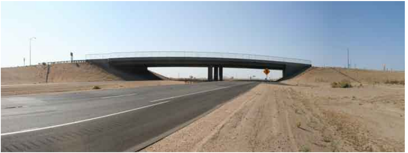
California City SR 14 Interchange Before Enhancements
