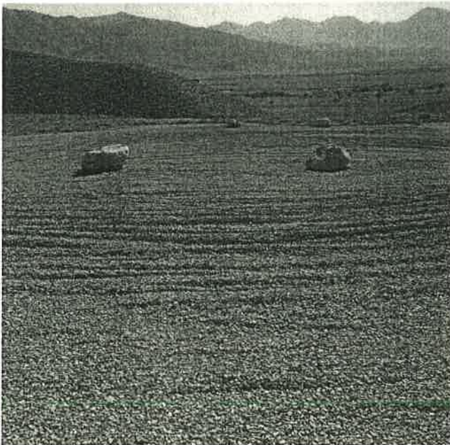
Improvements at Redding Cnyn OHV parking area
