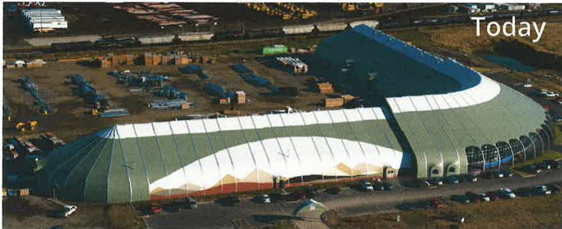
The Tedlar exterior today shows little difference to when it was installed.
