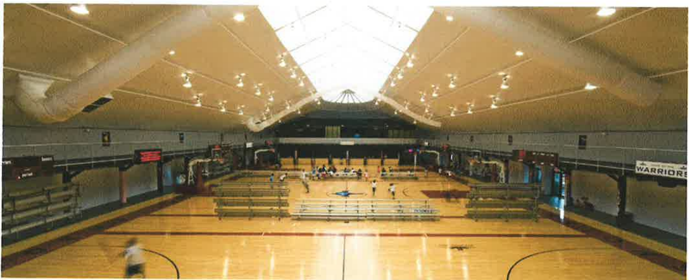
Sprung structure interior showing insulation system complete with tensioned interior membrane.
