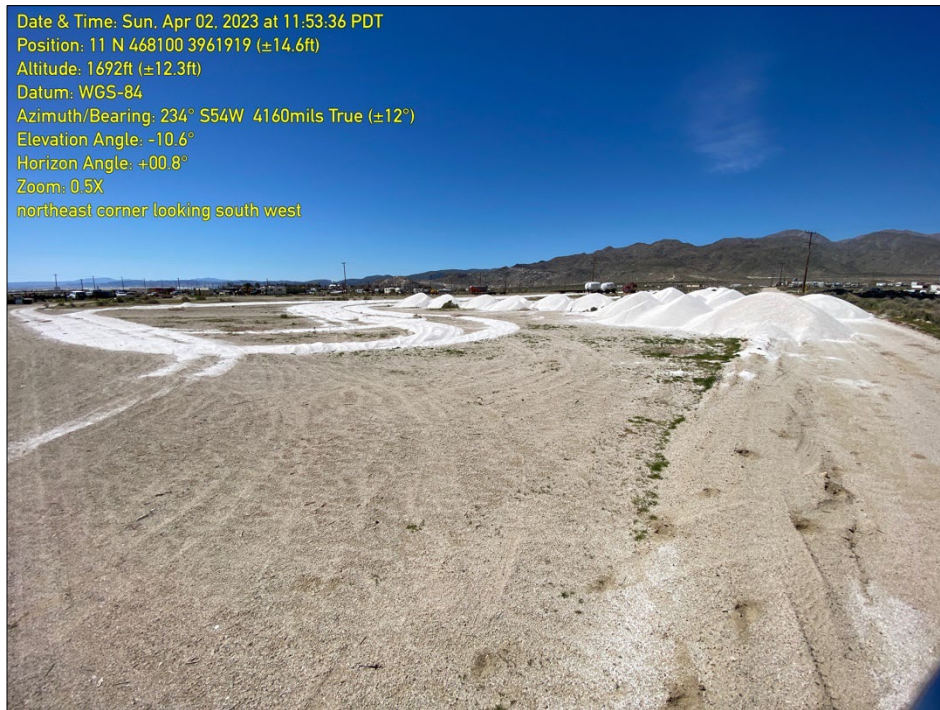
Photograph 1. Overview Site Photo – SBC Solar Project northeast corner, view to southwest. Denuded and in use for industrial raw materials storage.
