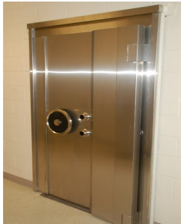
The Level 5 door of the Long-Term Storage Vault (same model used for each vault).
