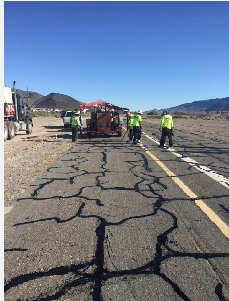
Shoshone Airport Crack Sealing
