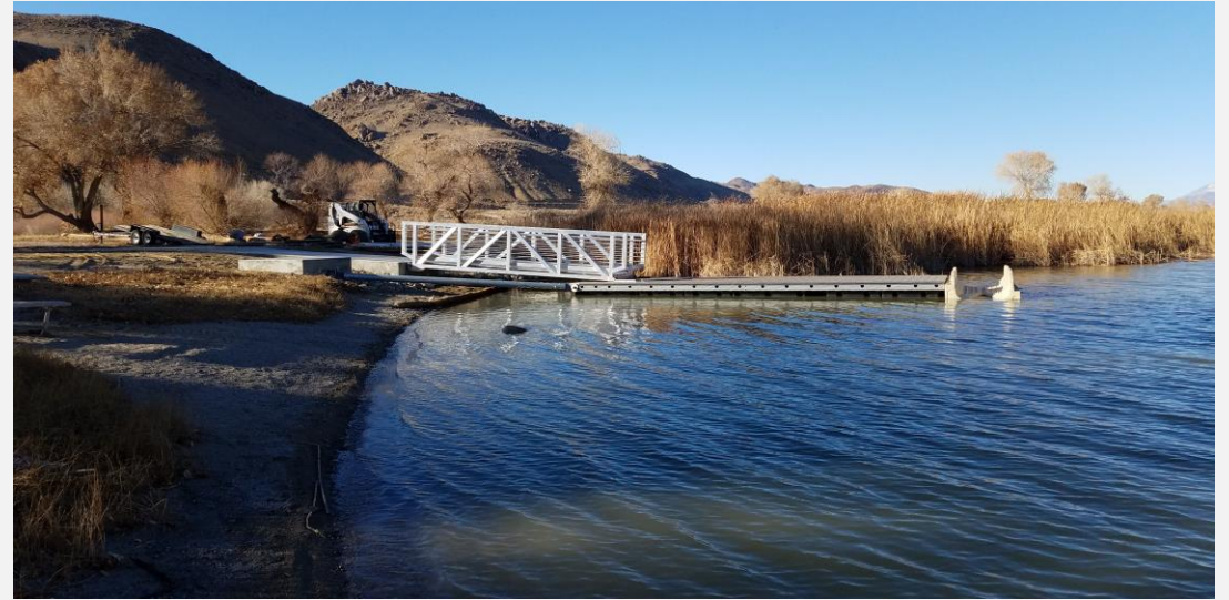
Lake Diaz ADA Boat Dock (Completed December 14 th 2022)
