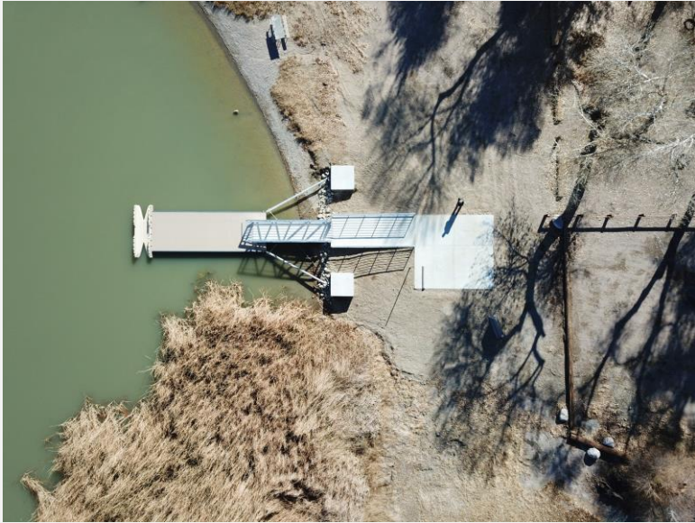
Lake Diaz ADA Boat Dock (Completed December 14 th 2022)
