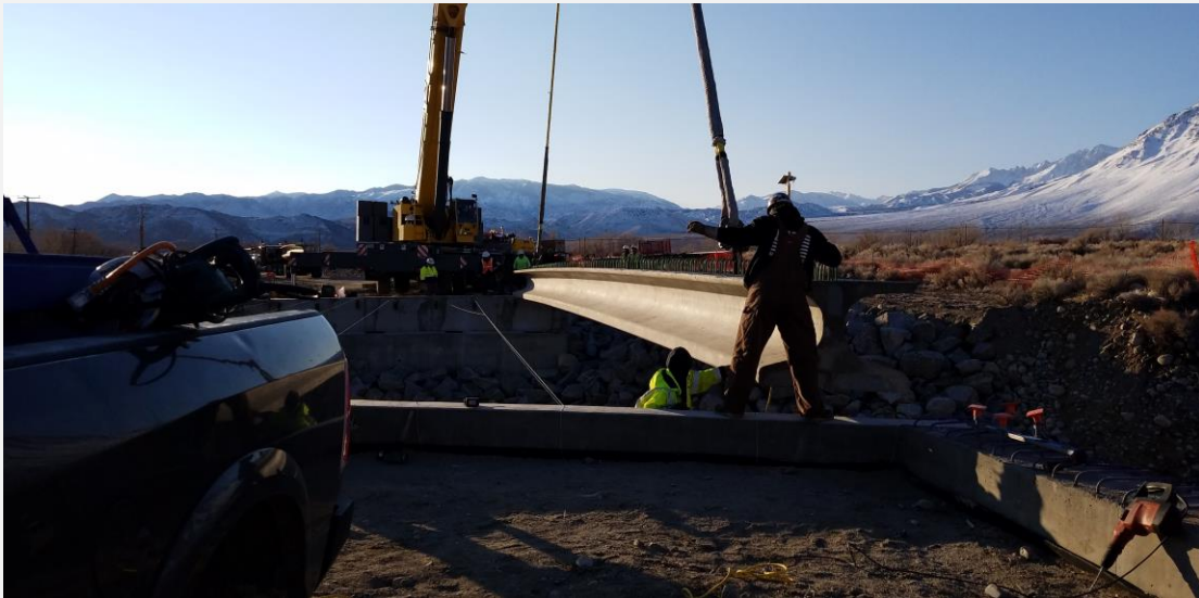
North Round Valley Bridge Girder Set (Project Ongoing)
