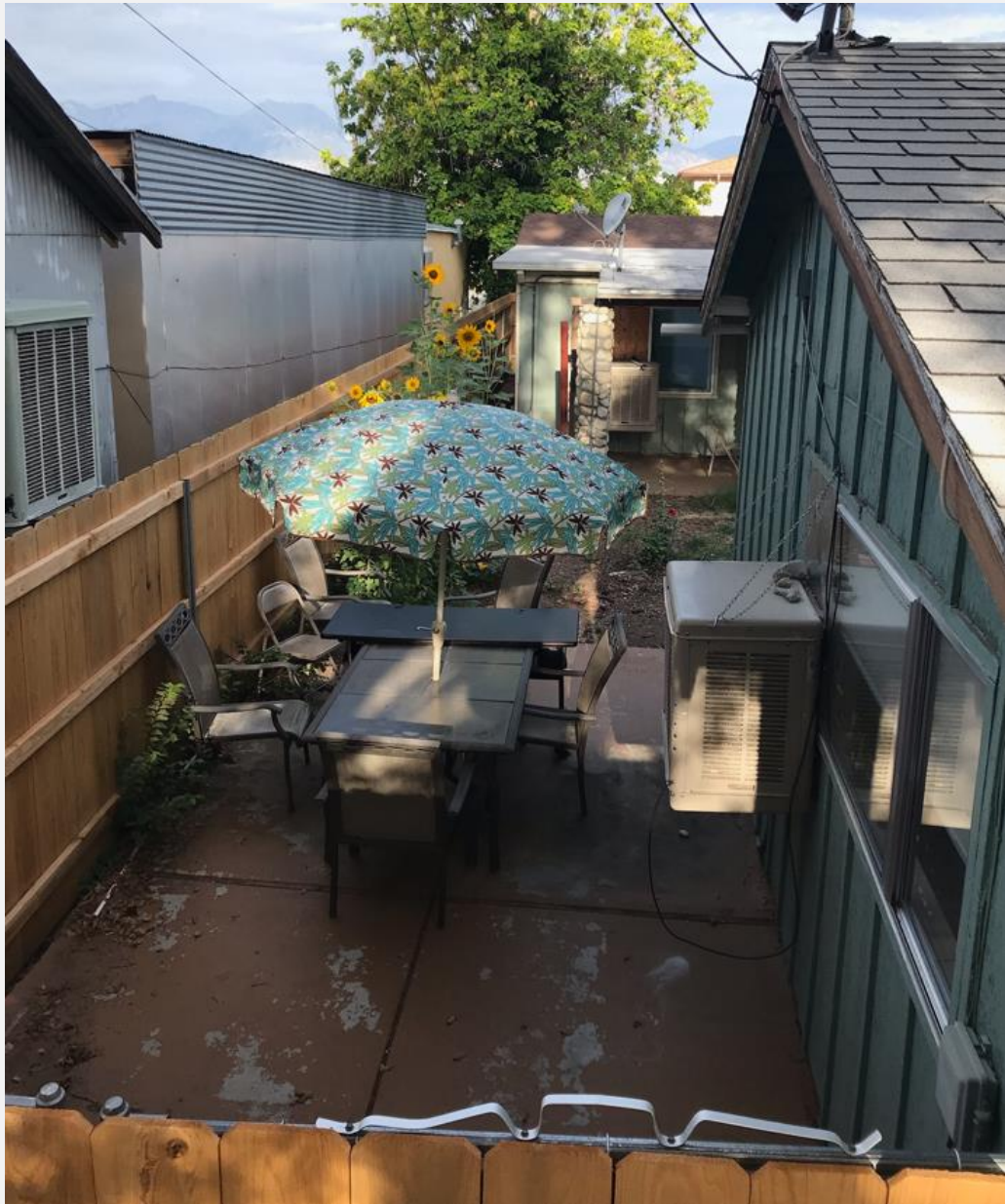
New Fence Installed at Progress House in Bishop.
