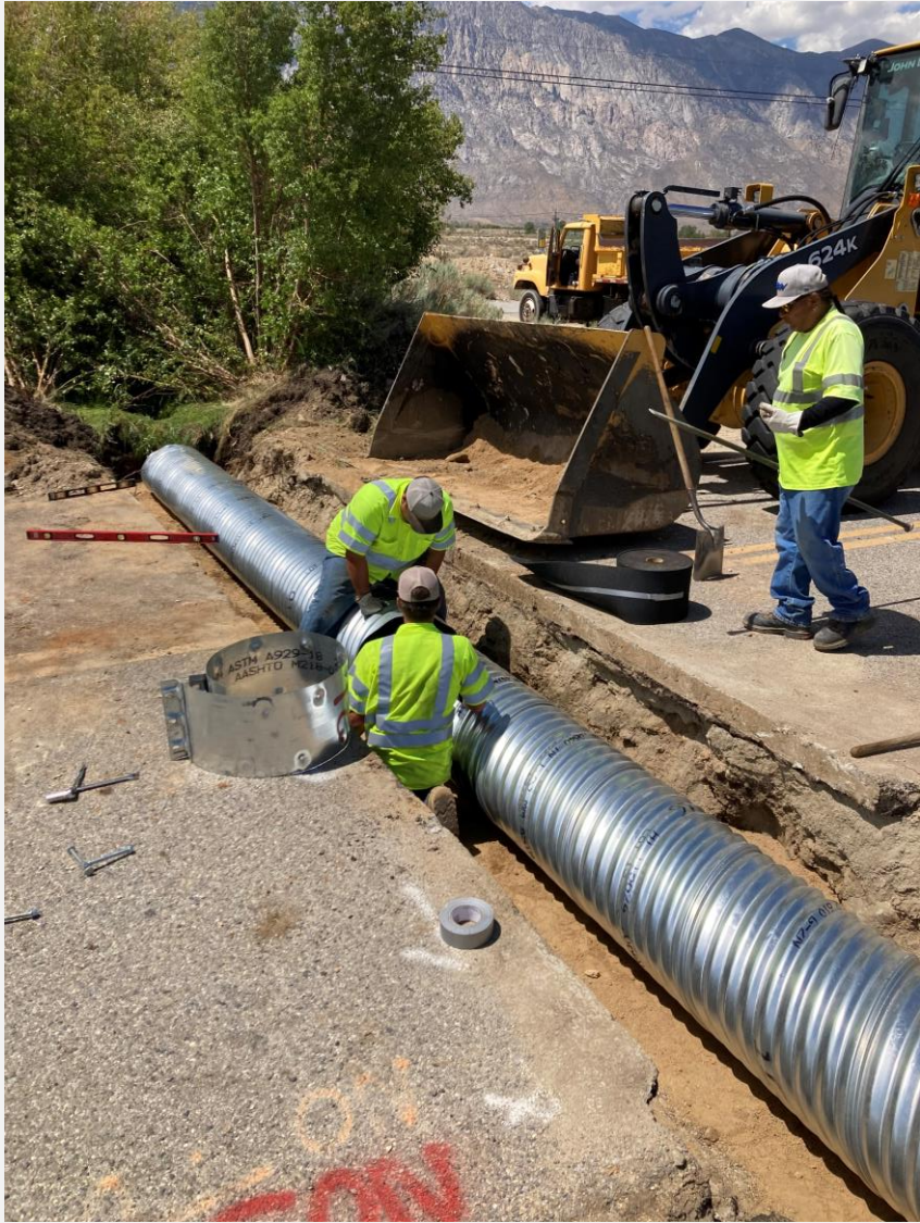
N Round Valley Road Culvert Replacement
