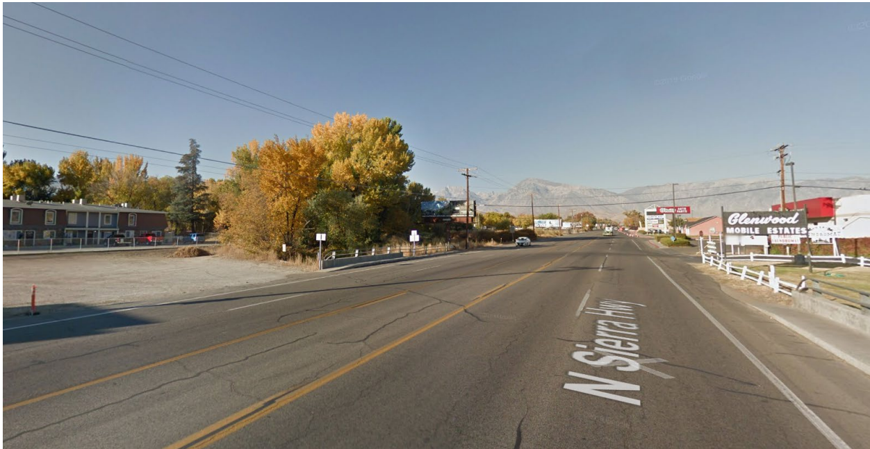
Figure 1 - Sidewalk gaps on north (right) and southbound sides of U.S. 395 at Bishop Creek Bridge.
