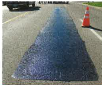
SKIN PATCH REPAIRS
