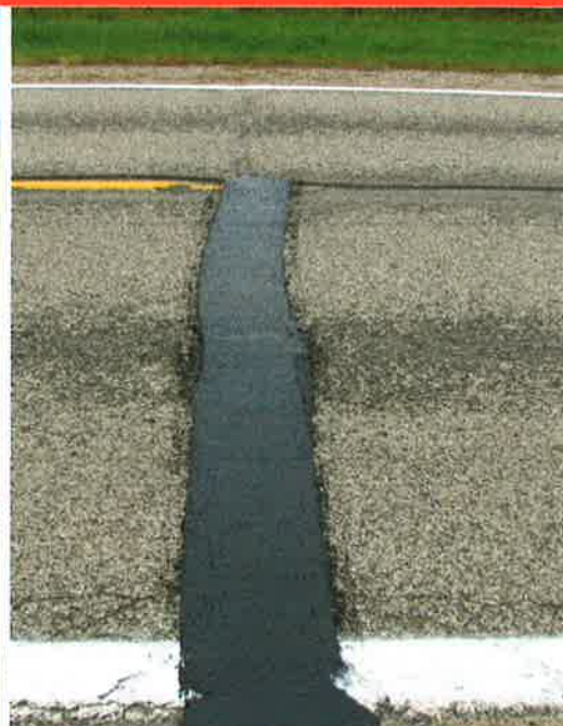
Filling Wide Cracks and Joints
