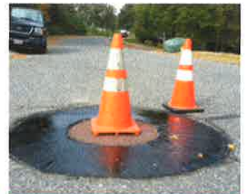
LEVELING MANHOLE COVERS
