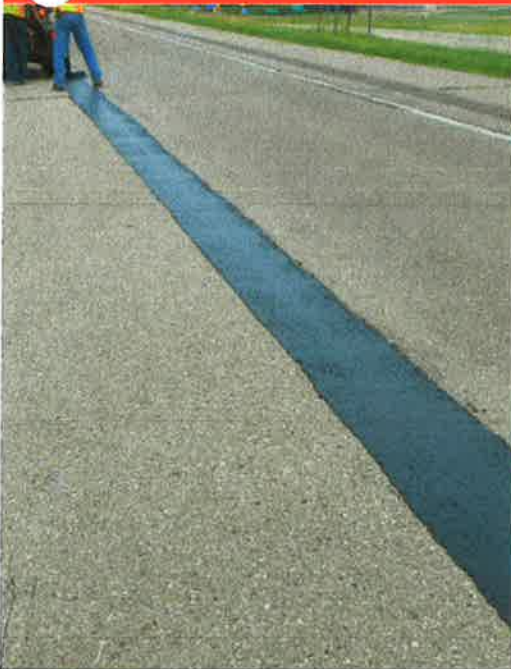
Repairing Deteriorated Longitudinal Joints
