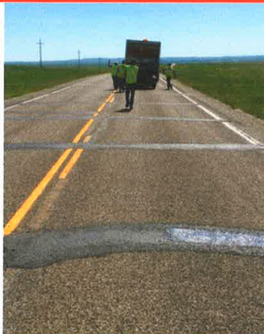
Leveling Depressed Thermal Cracks
