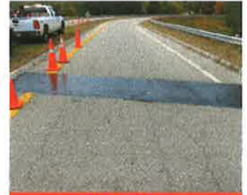
SEALING UTILITY CUTS
